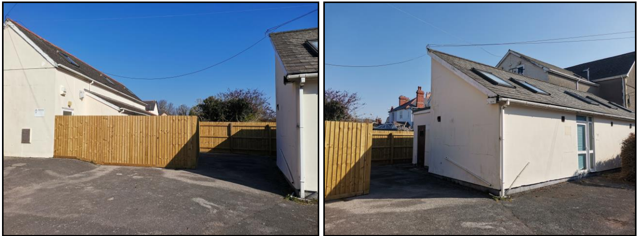
Existing Feather Edge Fencing Installed along property boundary
